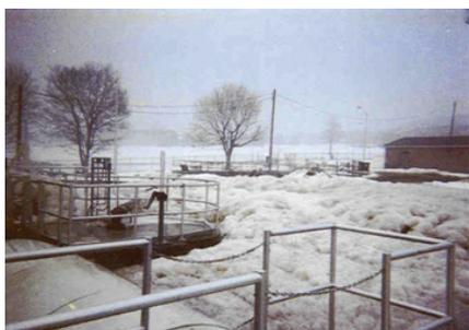
Fig. 1. Excess foaming from surfactants in wastewater.
